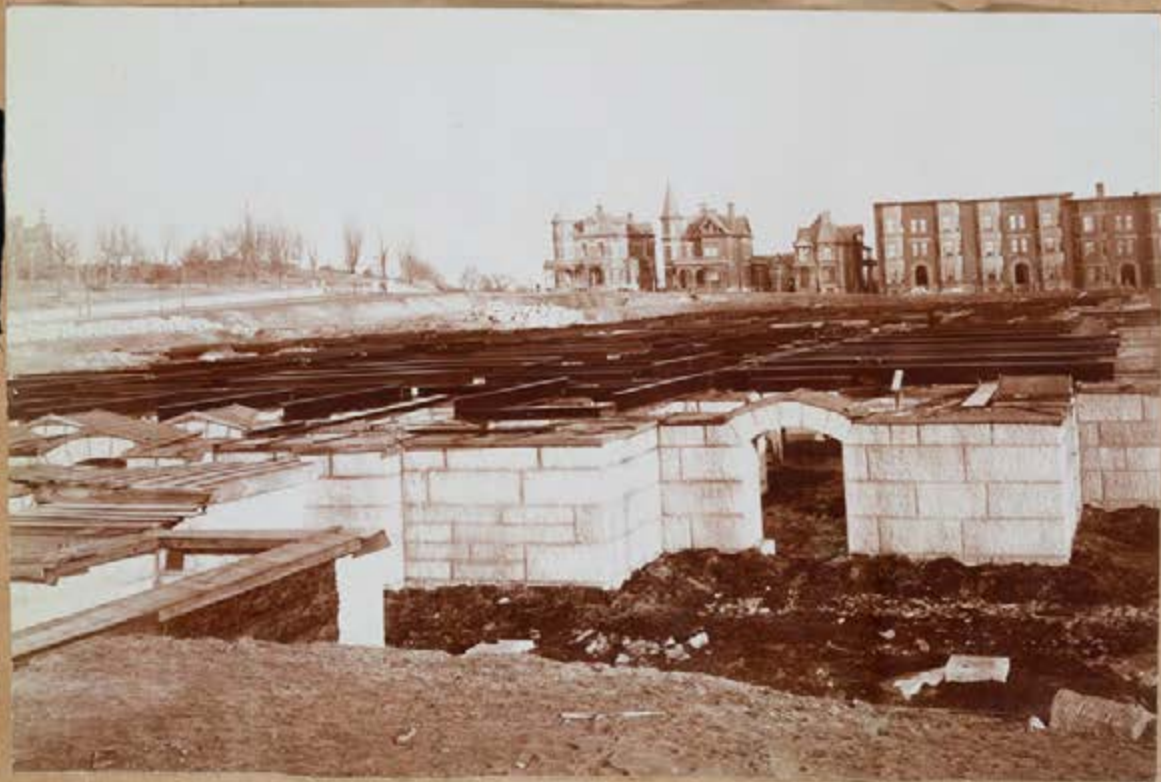
After steel for basement floor was in place
